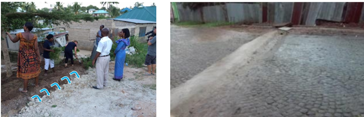
Figure 2: Establishment of gravel filled infiltration trenches is a simple way to help stormwater runoff find its way into the ground. Left: Stormwater management at single family parcel, Kibululu, Mbezi River Catchment, Dar es Salaam. Runoff from neighboring road that use to cause flooding and erosion on the parcel is now diverted into the ground. The family may afterwards use the systems for cropping of vegetables. Right: In Addis Ababa many soil roads are converted into cobblestone roads, but the conventional drainage systems add to problems with downstream flooding. Instead, we developed a drainage principle based on gravel filled infiltration trenches positioned across the hill to trap the runoff as it flows downhill.
